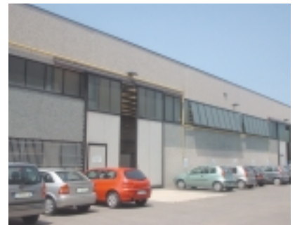
Bologna Technical Support Center
